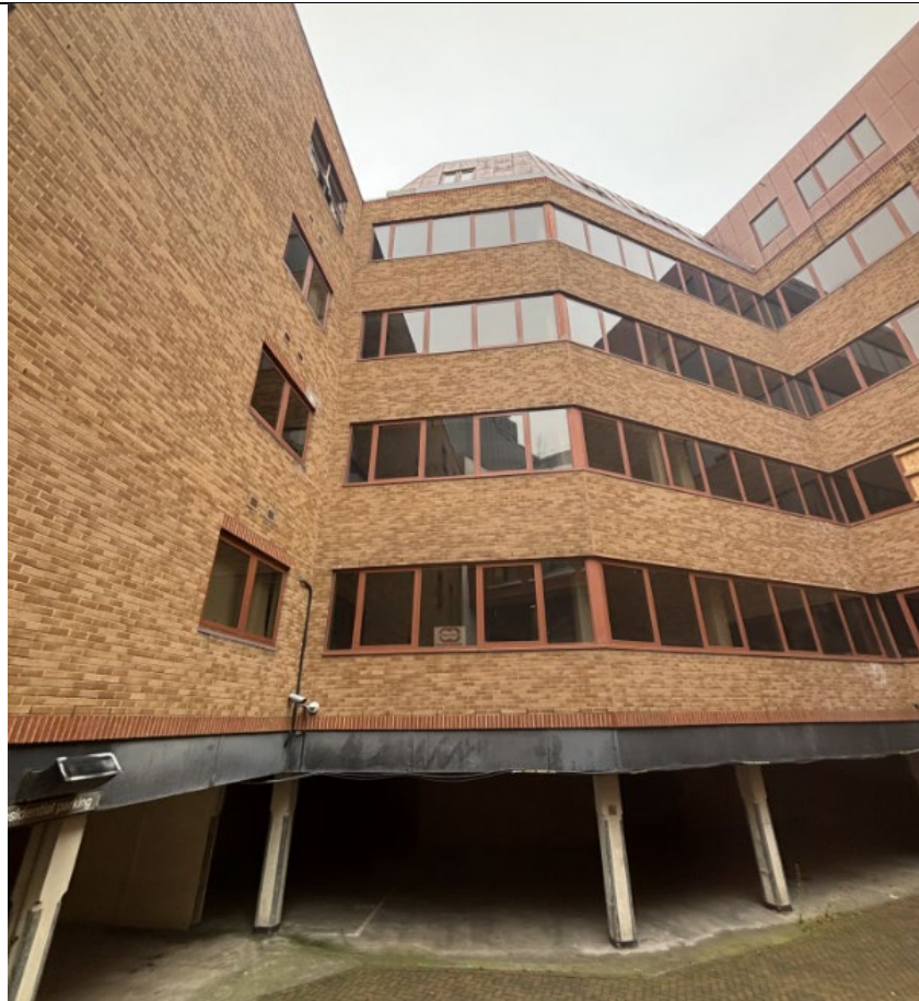
View of building from rear courtyard
